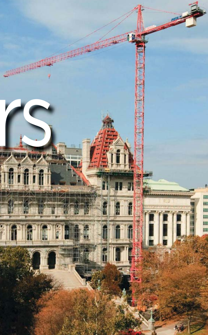
Photo courtesy of Consigli Construction.
