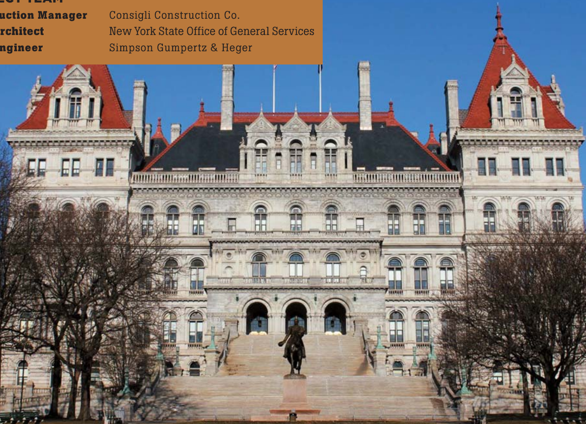
Photo courtesy of Consigli Construction.
