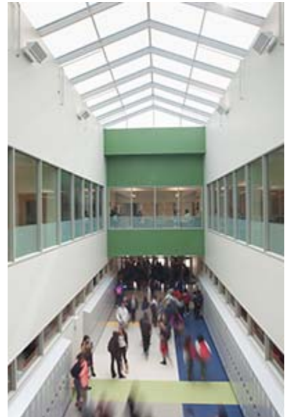
Skylights line Methuen High School's new entryway, introducing plenty of natural light into the space. Photo Credit (all): Finegold Alexander & Associates
