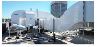
HVAC systems work by taking a percentage of recirculated interior air mixed with fresh air which, together, travels through a filter before being released into a building. These filters get dirty over time, collecting dust, debris and other airborne particles.
