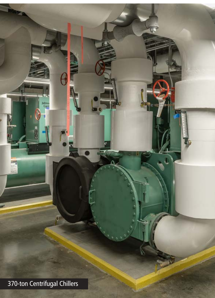
Primary Chilled Water Piping Distribution Header to Systems Heat Exchangers & Free-Cooling
